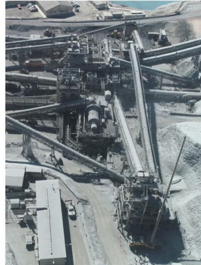
Candelaria plant pebble crushing circuit
